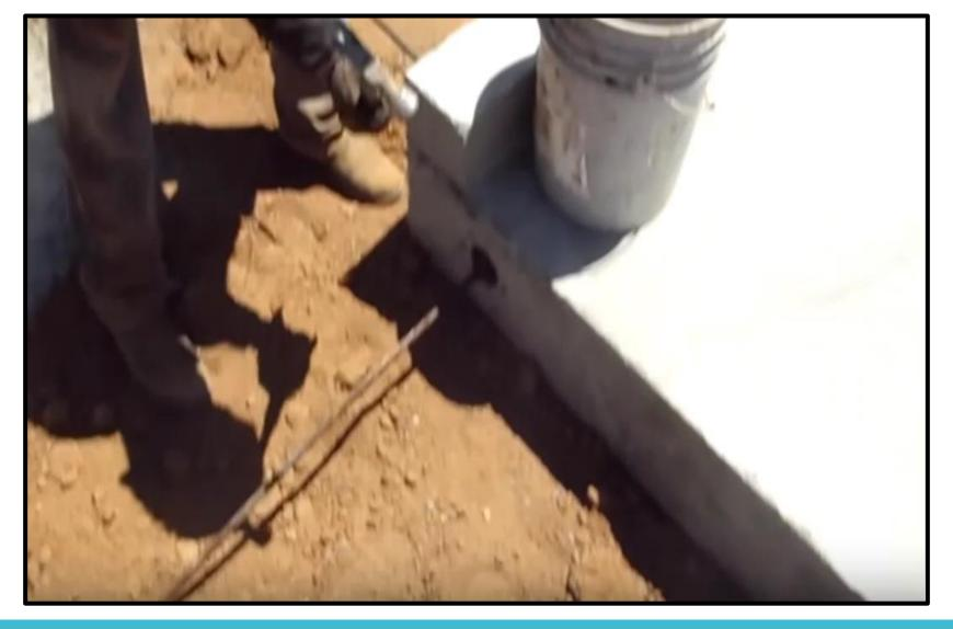
Pulling or stressing the steel cables squeezes the slab together preventing cracks in the foundation.
