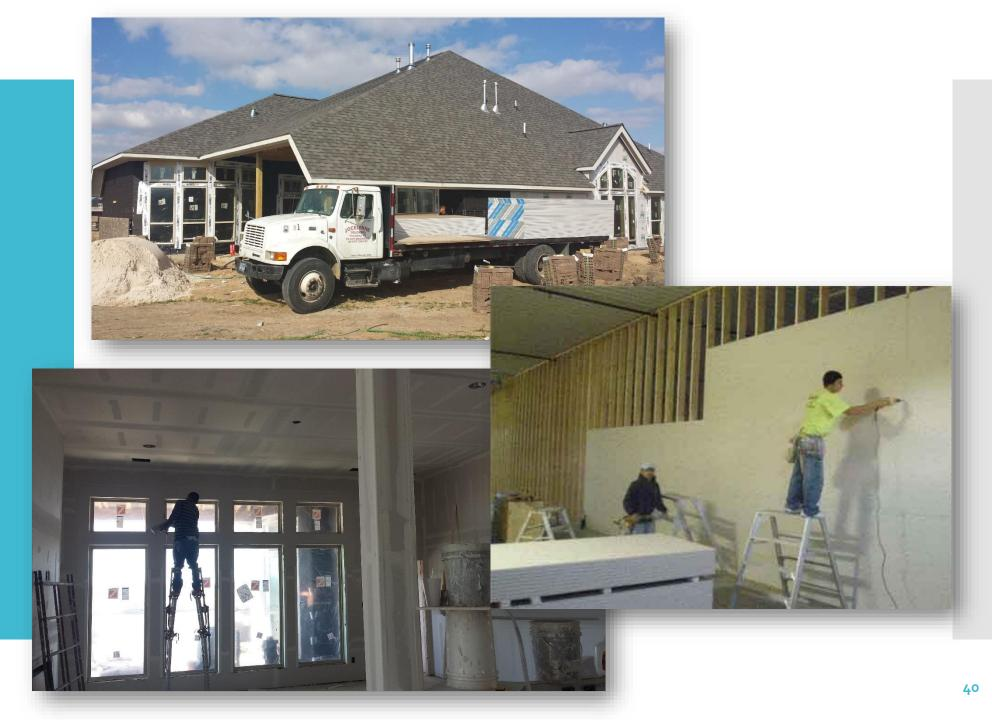
Sheetrock is a milestone because all the mechanicals in the walls must be completed and insulation must pass a third-party inspection.
