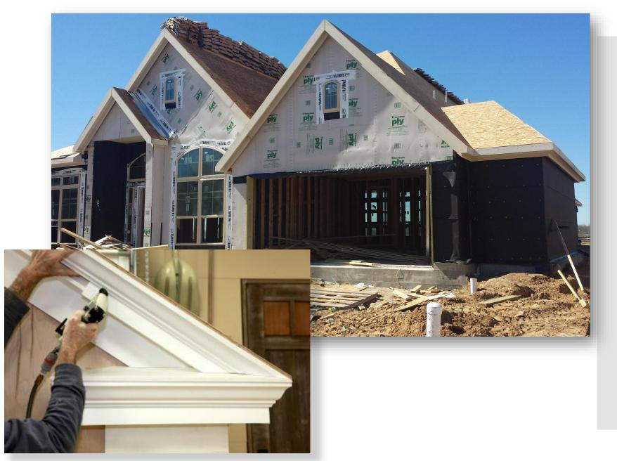
After the cornice stage the roof is decked with OSB (oriented strand board) to prepare it for shingles.
