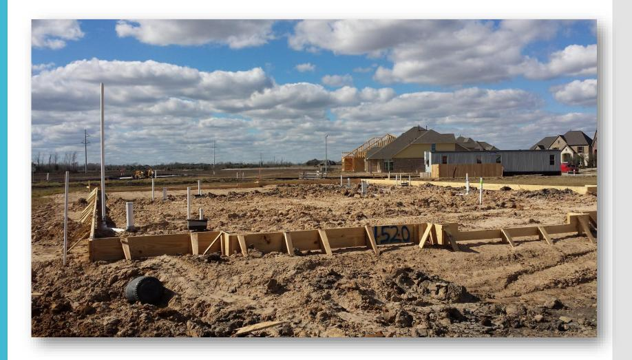
Piping, risers, tub buckets, and PEX water service to islands are in place prior to concrete.
